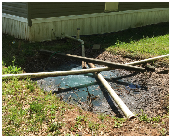
Straight piping sewage to ditch behind home in Lowndes County, Alabama. Photo Credit: DOJ/Civil Rights Division
